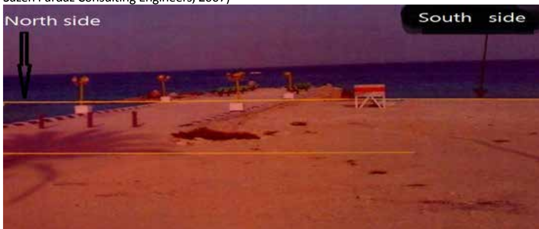
Figure 6 , Sedimentation manner on the southern coast of Simorgh Hotel's Pier (Source: Sazeh Pardaz Consulting Engineers, 2007)
